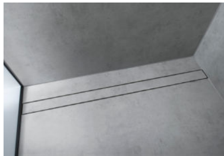
Rain Drain Rock
